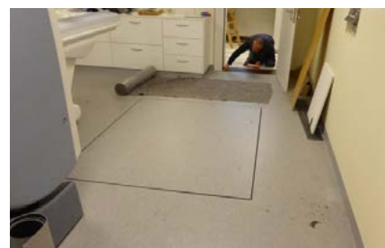
Level incorporated floor scale
